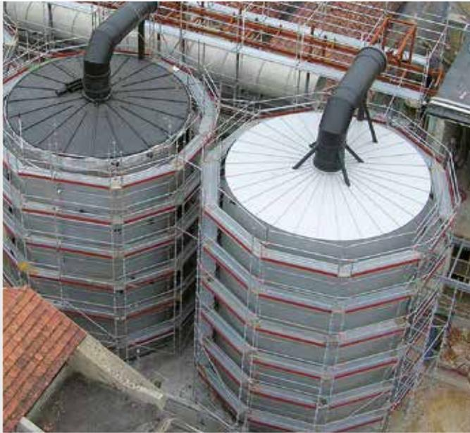
Air purification system, Spain. Material: HD-PE
