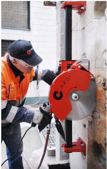
Cutting a reinforced concrete wall with the DV PE400-1500
