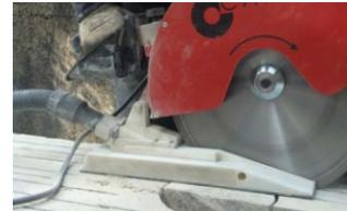
Dry cutting in reinforced concrete
