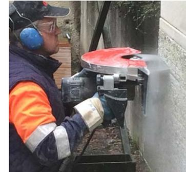
Wet cutting in reinforced concrete
