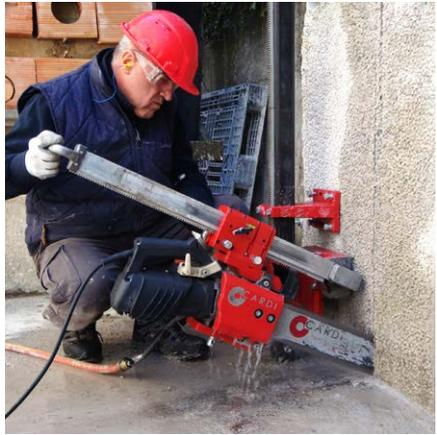
Finishing of a vertical cut in a reinforced concrete wall, going flush to the floor, with the DV CD35-1500
