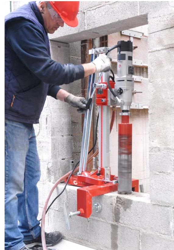
FLUSH TO THE WALL DRILLING (OR FLOOR) AND INTO THE CORNERS
