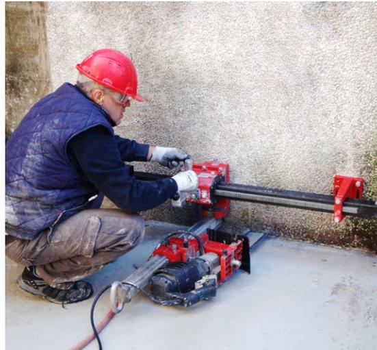
Flush cutting in a reinforced concrete wall with the DV CD35-1500
