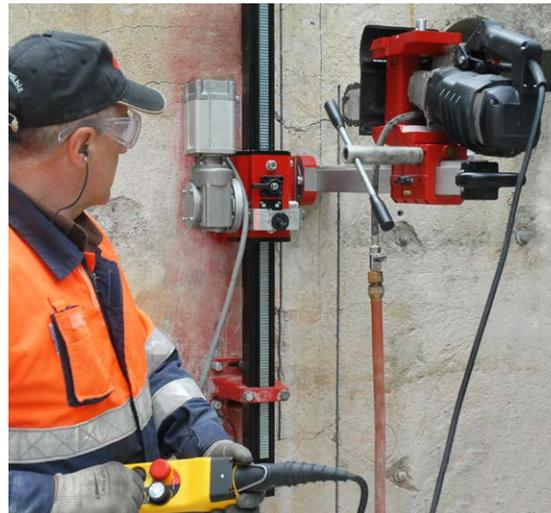
Cutting with the DV CD35-1500 using the semi-automatic feeding system DA VINCI SERVO (see pag. 21)
